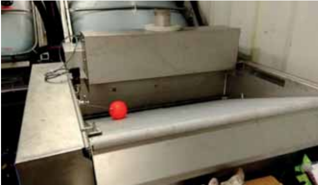
Picture 4: The purpose of the belt filter is to separate excessive water from the sludge.
